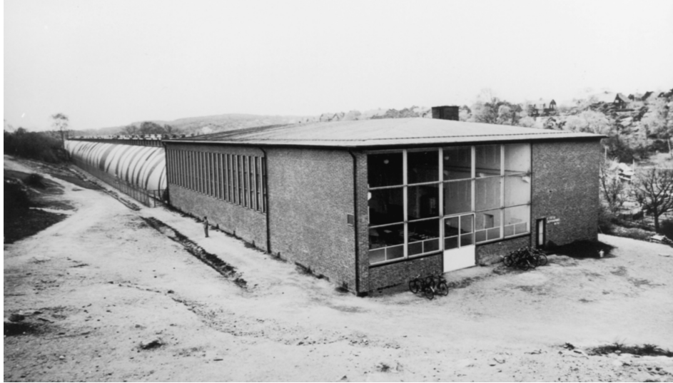
The Swedish State Shipbuilding Experimental Tank began operation in 1940. Note the war-time camouflage painting of the arched roof over the tank. (Photo: SSPA)
